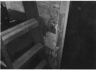
There were moisture stains on the ceiling of the garage around the boiler flue pipe penetration that appeared to be from a past or present roof leak. It was not possible to determine if the roof was currently leaking and all stained areas appeared dry at the time of this inspection. Consult with the seller for additional information and have the roof serviced as needed.
