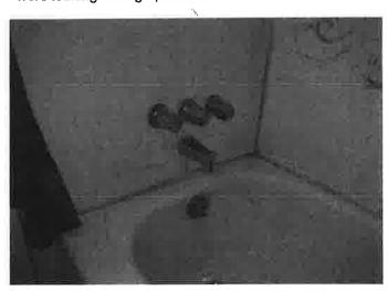
The master bath stall shower cold water faucet was leaking at the stem during operation.
