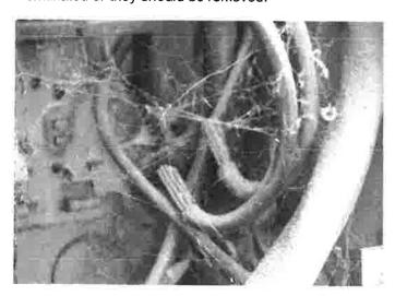
• There was an electrical circuit breaker that had been wired incorrectly to two circuits. This condition was also observed at the neutral bus bar. This is commonly referred to as double-lugging and should be repaired by a licensed electrician.
